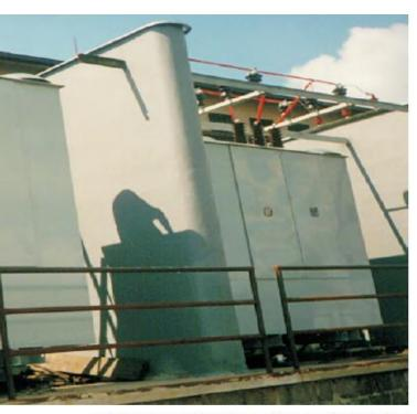
Traction transformer in outdoor cubicle version 38T-23SF-184/83 5,3MVA - substation Opočinek
