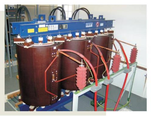
Traction transformer 1100 kVA, 22/0.65 kVA in vault of trolley bus substation
