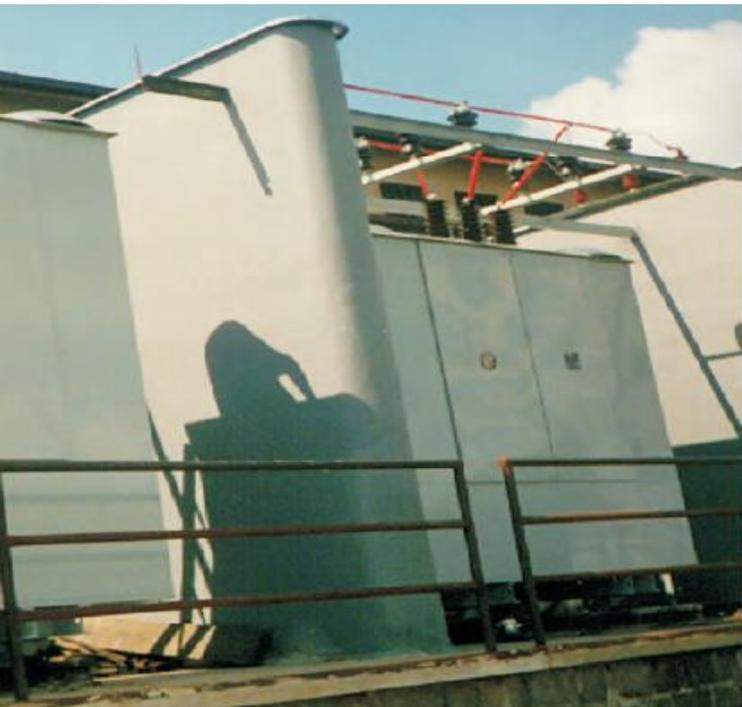
Traction transformer in outdoor cubicle version
