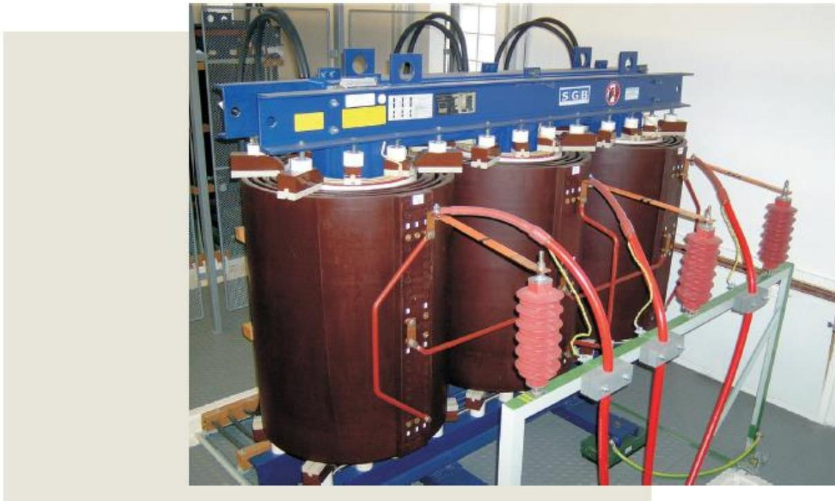
Traction transformer 1100 kVA, 22/0.65 kVA in vault of trolley bus substation
